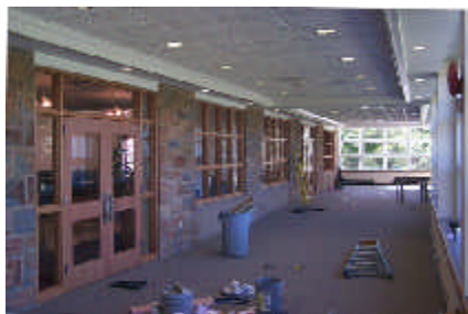
HUB dining expansion as seen during the construction phase
